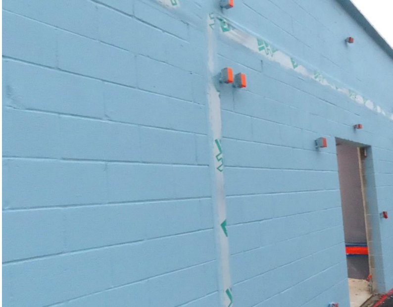
Installing liquid & peel and stick on CMU walls
